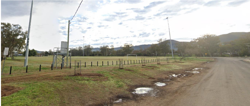
Example of damage caused by vehicles parking in informal areas (Gipps Street Sporting Fields).
